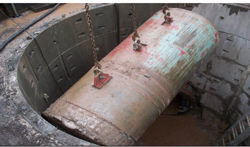
TUNNELLING MACHINE RECOVERY
