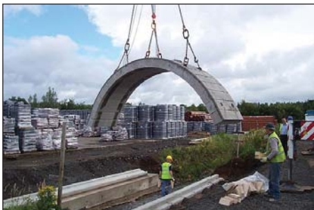
Flexible arch system during lifting
