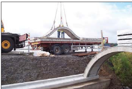
Flexible arch system during lifting
