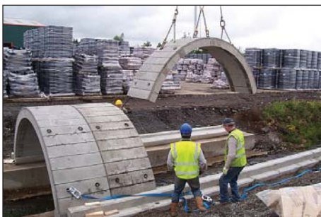
Arch system positioned on tapered seating units
